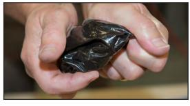
Mix the hardener and resin together for approximately 2-4 minutes by working the bag in your hands. The resin will start to warm up after 2-3 minutes of mixing. In winter, mix for 4-5 minutes.
