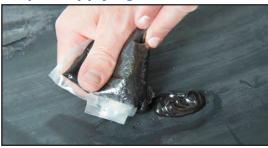
Cut an opening in the bag that suits the repair you are doing. For small spot repairs only cut a small hole in the corner. For larger repairs cut a bigger hole. Apply the resin to the damaged area by squeezing it out of the bag.
