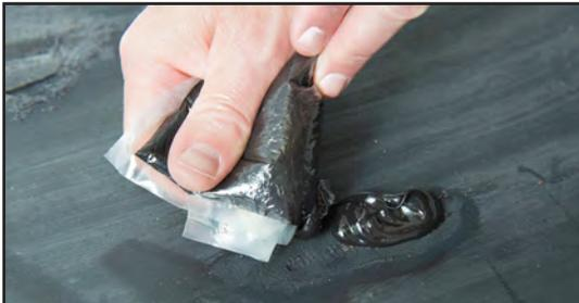
Cut an opening in the bag that suits the repair you are doing. For small spot repairs only cut a small hole in the corner. For larger repairs cut a bigger hole. Apply the resin to the damaged area by squeezing it out of the bag.
