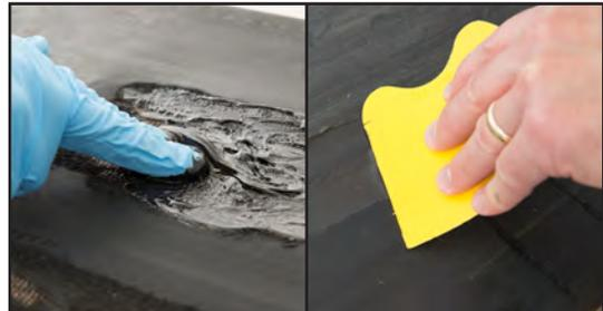
Work a thin layer of Eli-Flex into the prepared surface with your fingers. Continue spreading Eli-Flex using a spatula or any other flat-edged tool. Working time is approximately 20-30 minutes. After approximately 45 minutes the resin will gel, and after 120 minutes it will set. It is now ready for belt operation, but will take 8-10 hrs to reach full strength.
